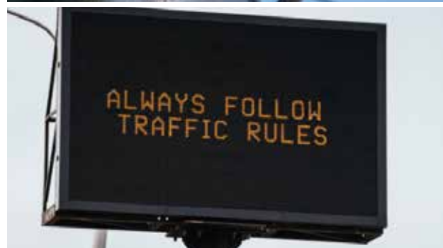
Figure-15: Public Address System (left) and Dynamic Message Sign Boards (right) (BSCL, 2022)
