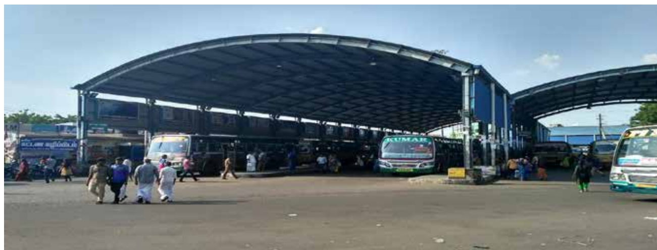
Figure 5 – Views of Old Chathiram Bus stand Source: Detailed Project Report
