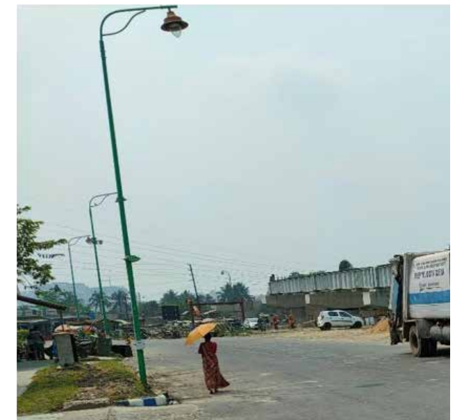
Figure 9: Street lights using energy from the Bio-methanation plant Source: Authors energy obtained from the bio-methanation plant.
