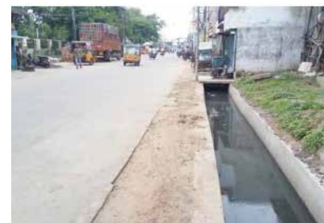
Figure - 4 Uneven Pedestrian Surface with Obstructions
